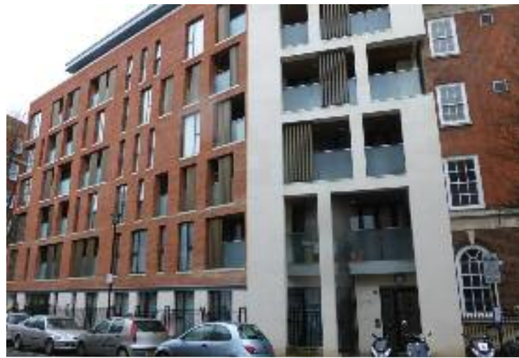
21 homes at Lavington Mansions, Ogle Street, were completed last year.
