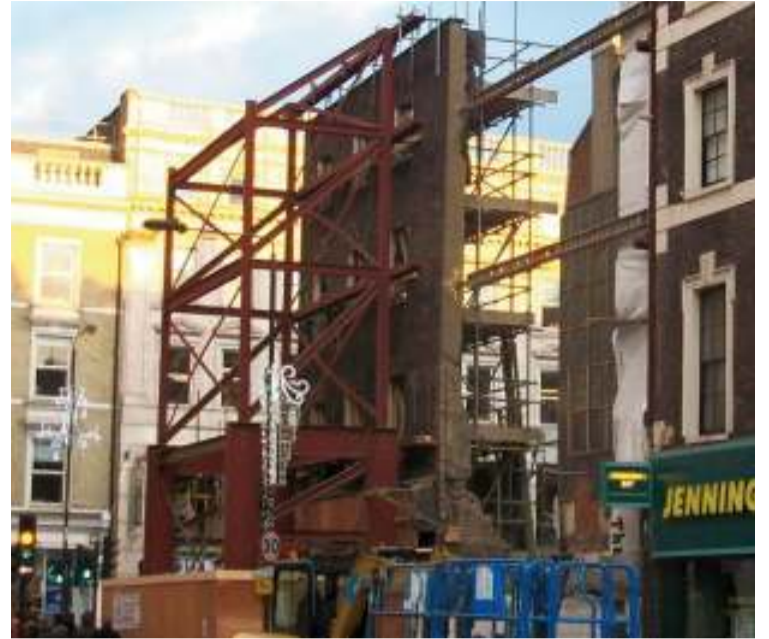
Facade of 1-3 Goodge Street held up by girders before it was demolished.
