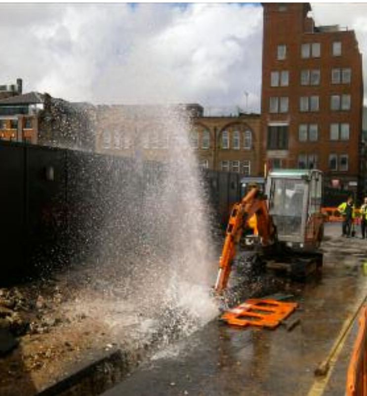
A mechanical digger strikes a water main on Cleveland Street during work to lay cabling. See "Running water everywhere" page 4.
